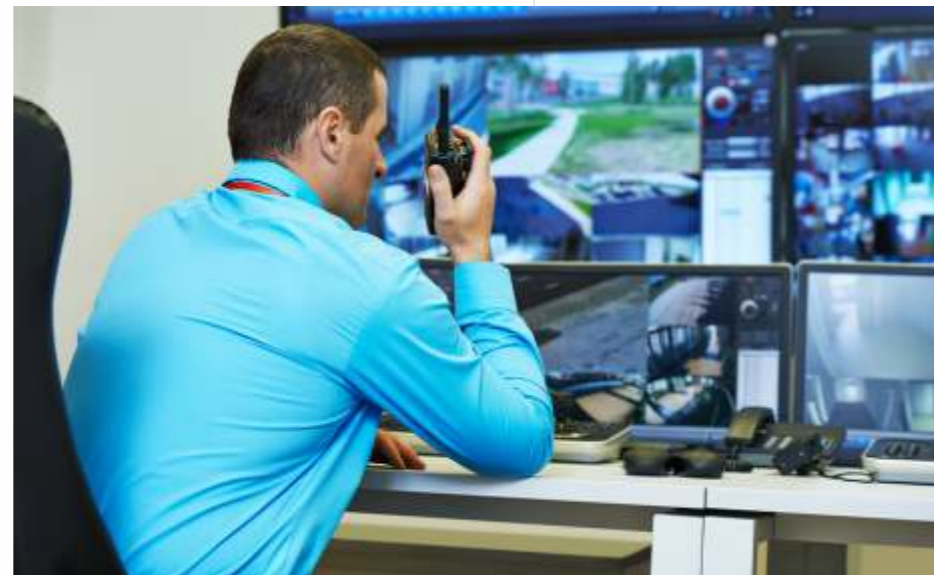
Health monitoring of the surveillance system to reduce device or component failure rates.
